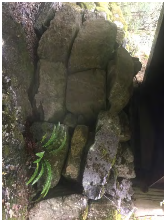
Right Bank Abutment when facing downstream
